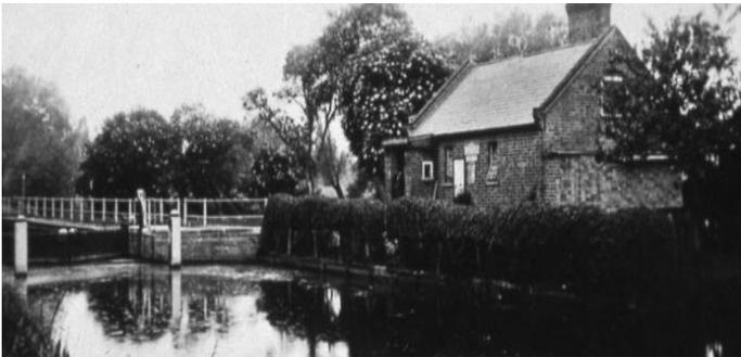
**Carthegena Lock** was built as a turnpike in 1741 and rebuilt as a pound lock in 1767/8 in Broxbourne Gull, which was an existing flood channel, separate from, but roughly parallel to Broxbourne Mill Stream. Whilst not a man-made channel, it may have been improved over the years. The lock is 17.5 miles from Bow Creek and has a drop of about 5 feet. Directly behind the lock is Carthegena Weir, part of a fishery which also includes two lakes and a section of the Old River Lea.
